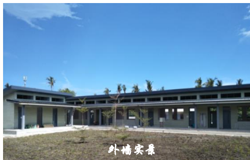
Real Picture of External Wall
