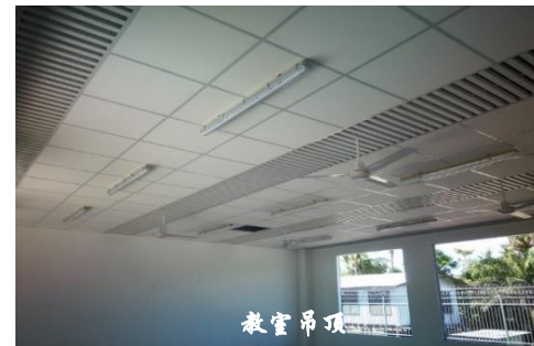
Real Picture of Classroom Ceiling
