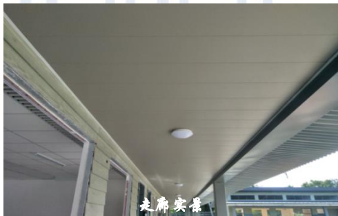
Real Picture of Corridor
