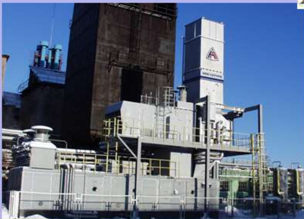
Gas turbine power plant with a capacity of 2.5 MW recovery boilers
