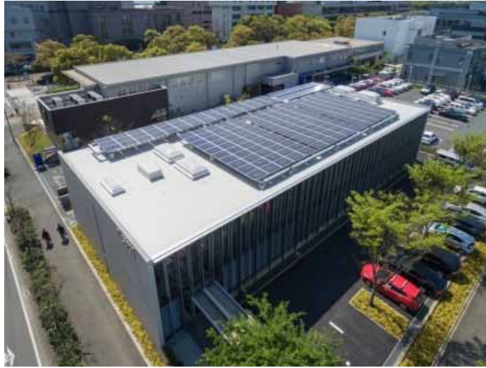
Devices on the roof
