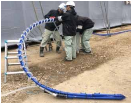
Geothermal heat collecting pile (During construction)
