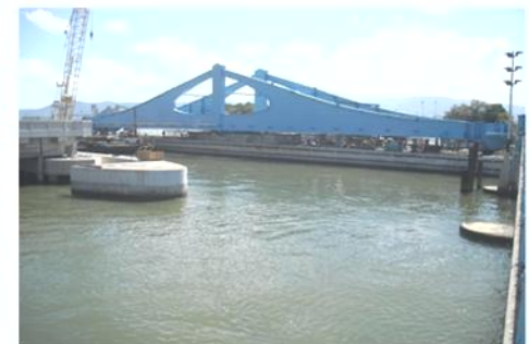
Jambatan Putar Perai
