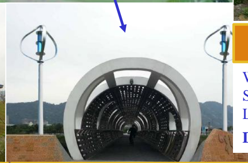
Long kiln bridge 700W wind turbines 2sets
