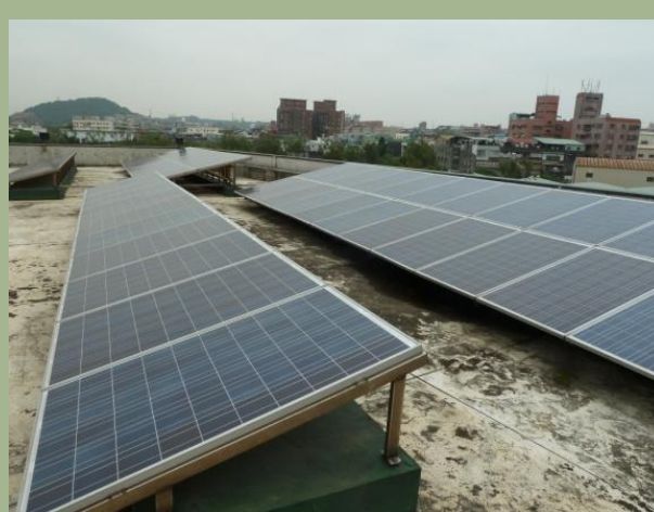
Solar power system in Visitors center (Crystalline silicon 15.18kWp)
