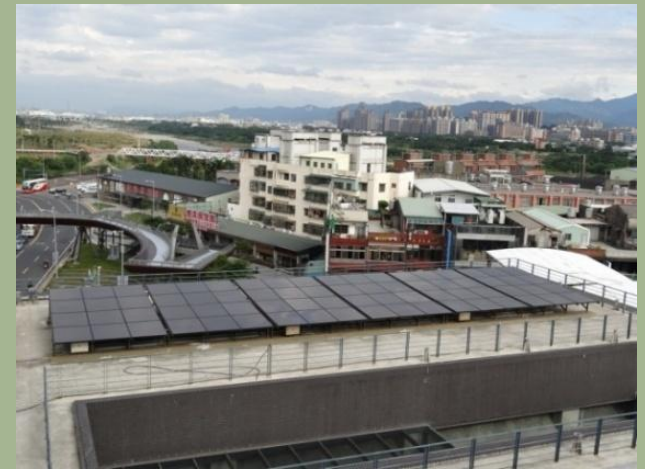
Solar power system on Museum's rooftop (Film 20.88kWp)
