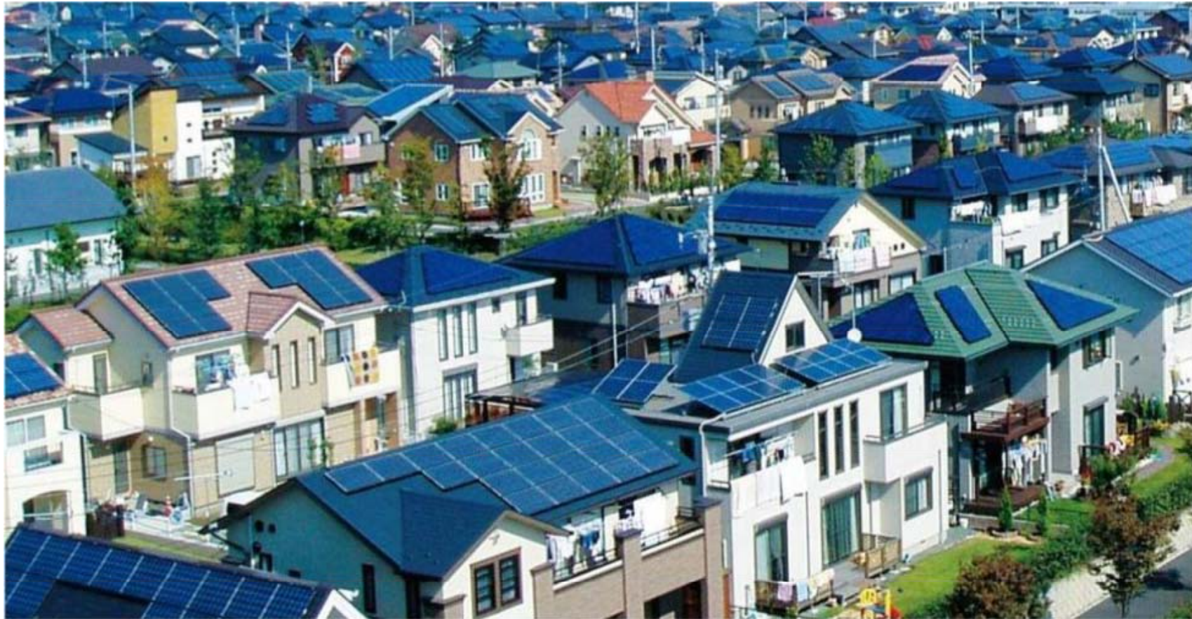
Ota City Demonstration Site
