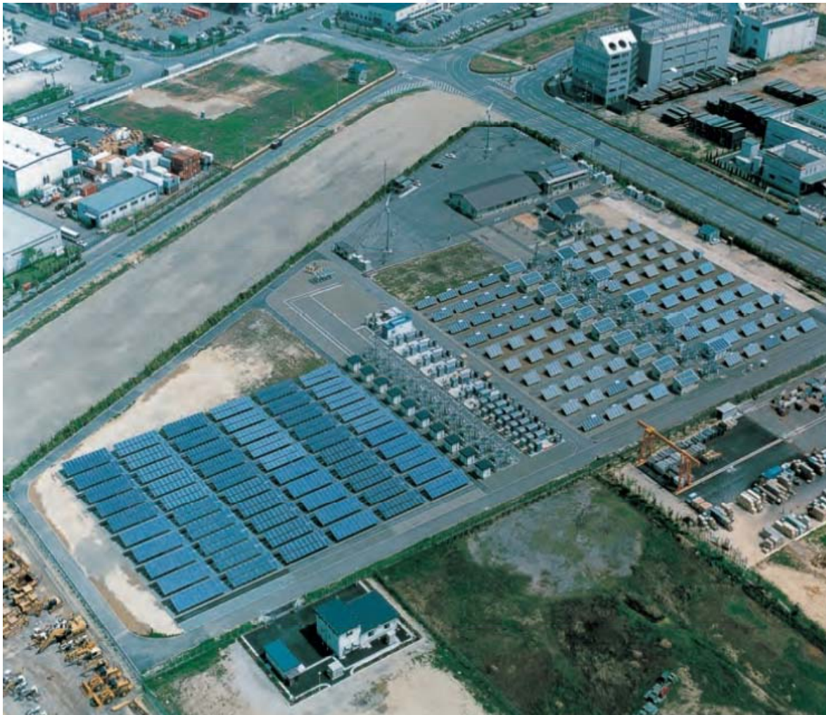
Rokko New Energy Test Facility (Kansai Electricity Power Co.)
