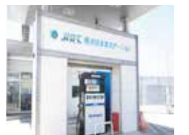
The JHFC Yokohama-Asahi Hydrogen Station
